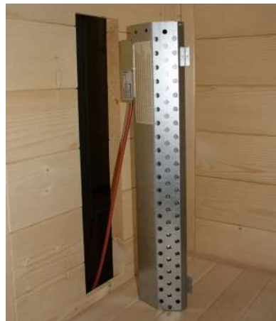
Fig. 2: Terminal box position
